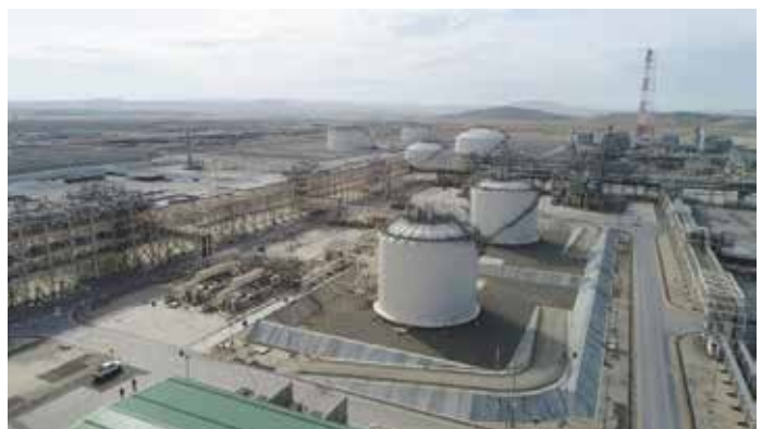
Azerbaijan, Sangachal Terminal Project - Mechanical Works, Electrical Equipment and Installation of Control-Measuring Devices
